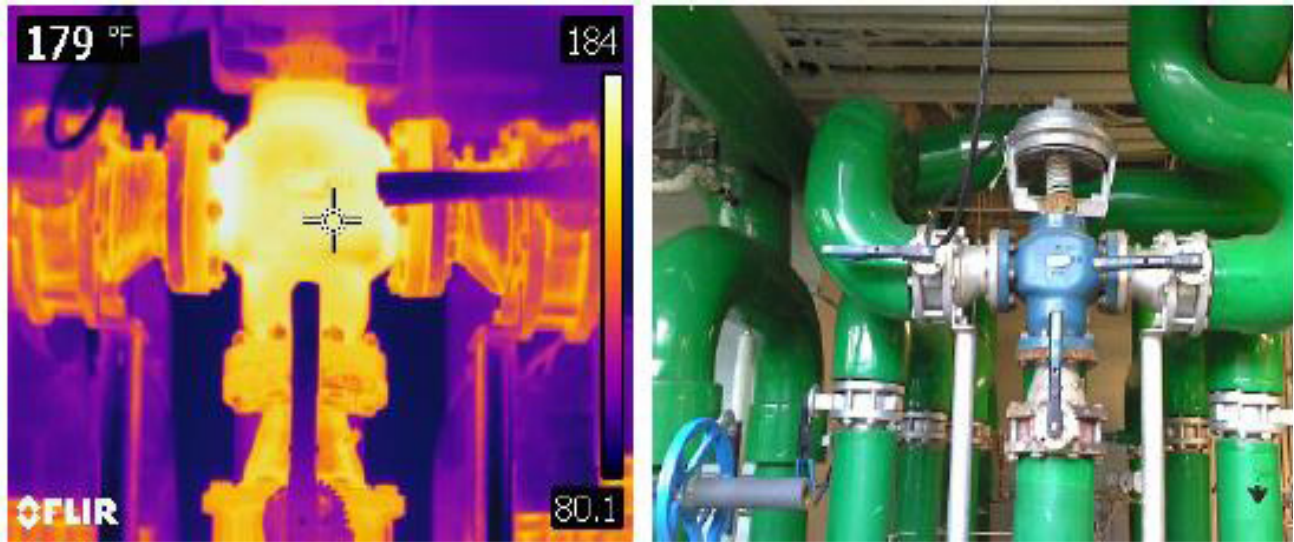
Bare heating valves in the boiler room of the Reynolds Museum
