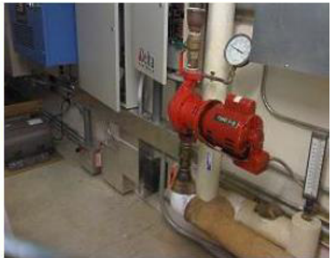
Figure 34 Conventional image of the same motorized heating pump.
