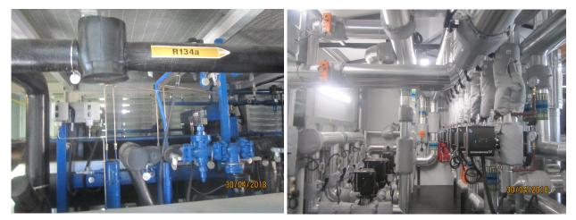
Photos: Air source heat pump system (above), with gas back up
