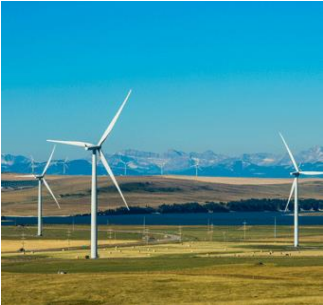
Figure 3 – IKEA’s Wintering Hills wind farm in Drumheller, Alberta (Canada). With 55 wind turbines, this farm could generate 88-MW, which is enough electricity to power 54 IKEA stores (IKEA Canada, 2018).
