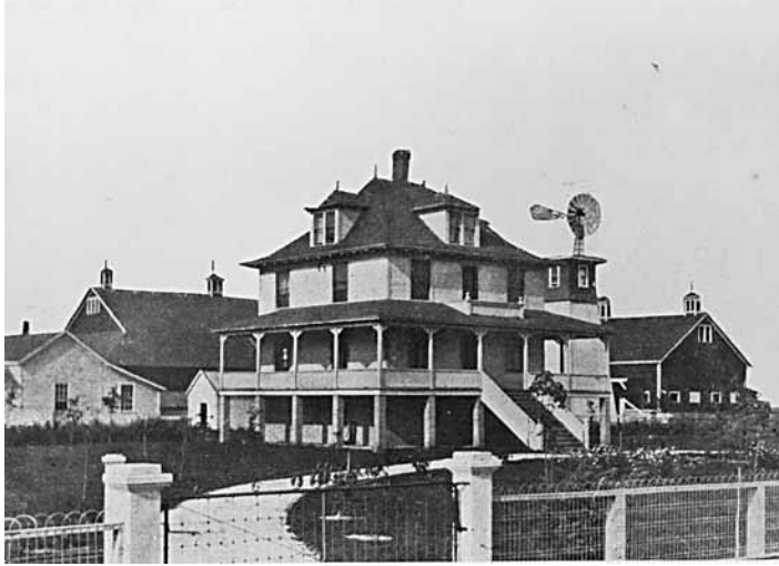
Figure 2.5 - Picture of Burns' Ranch manor house Manor house is in the centre of the picture with a barn visible behind the house to the right and a second house on the left, taken in 1908 (Delta Museum and Archives collection).
