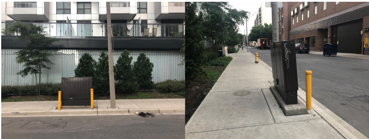
Figure 5. Existing above-ground equipment without aesthetic treatment, tagged with graffiti. Toronto, Ontario. June, 2019.
