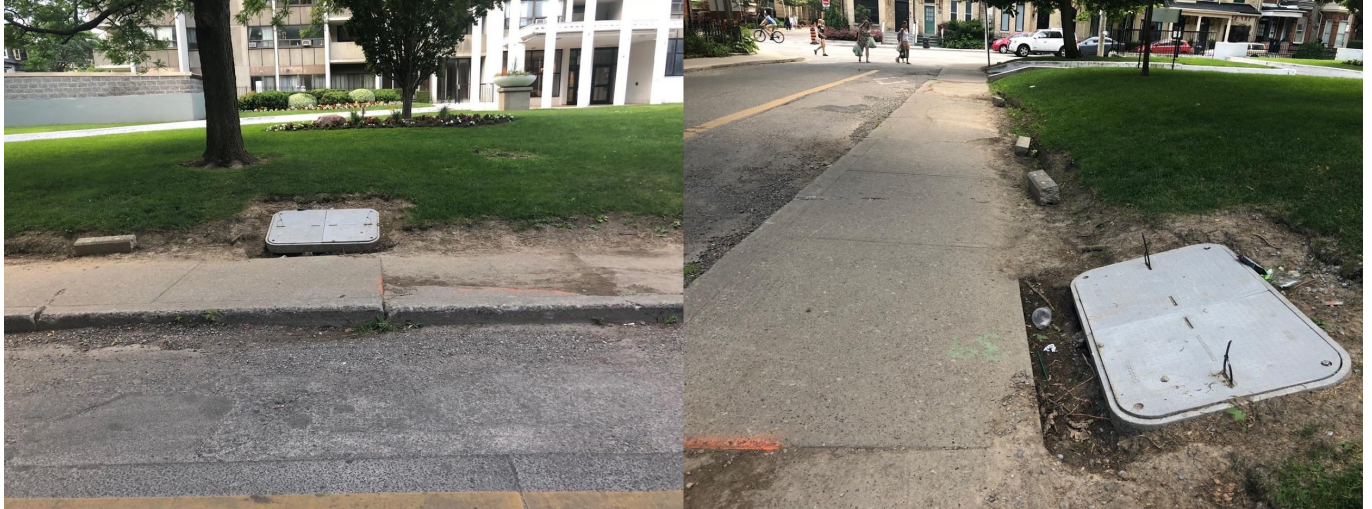
Figure 3. Grade level installations in a pedestrian zone. Toronto, Ontario. June, 2019.
