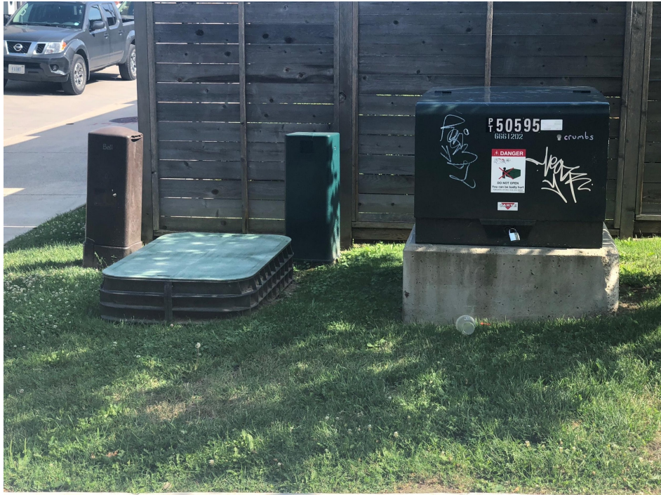
Figure 4. Clustering of equipment with no aesthetic treatment. Toronto, Ontario. June, 2019.
