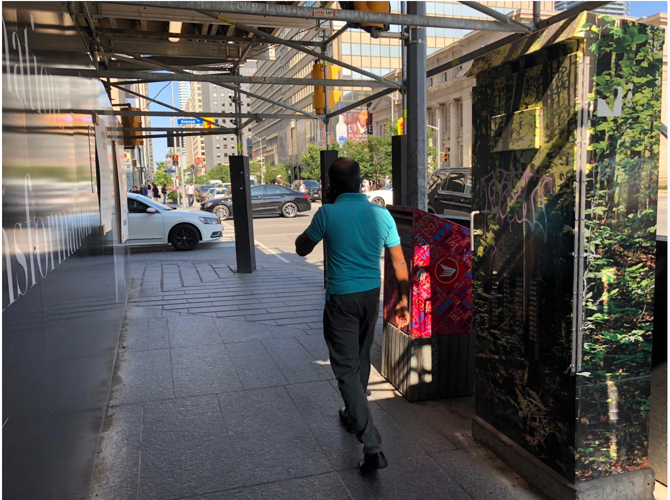
Figure 8. Above ground equipment with a 'natural' design applied as a decorative cover. Toronto, Ontario. June, 2019.
