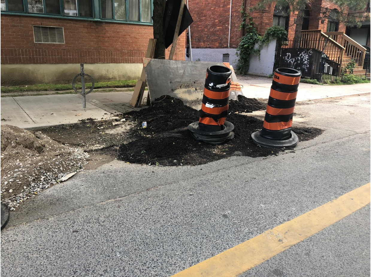
Figure 10. Image of temporary paving, awaiting resurfacing after maintenance/installation. Toronto, Ontario. June, 2019.
