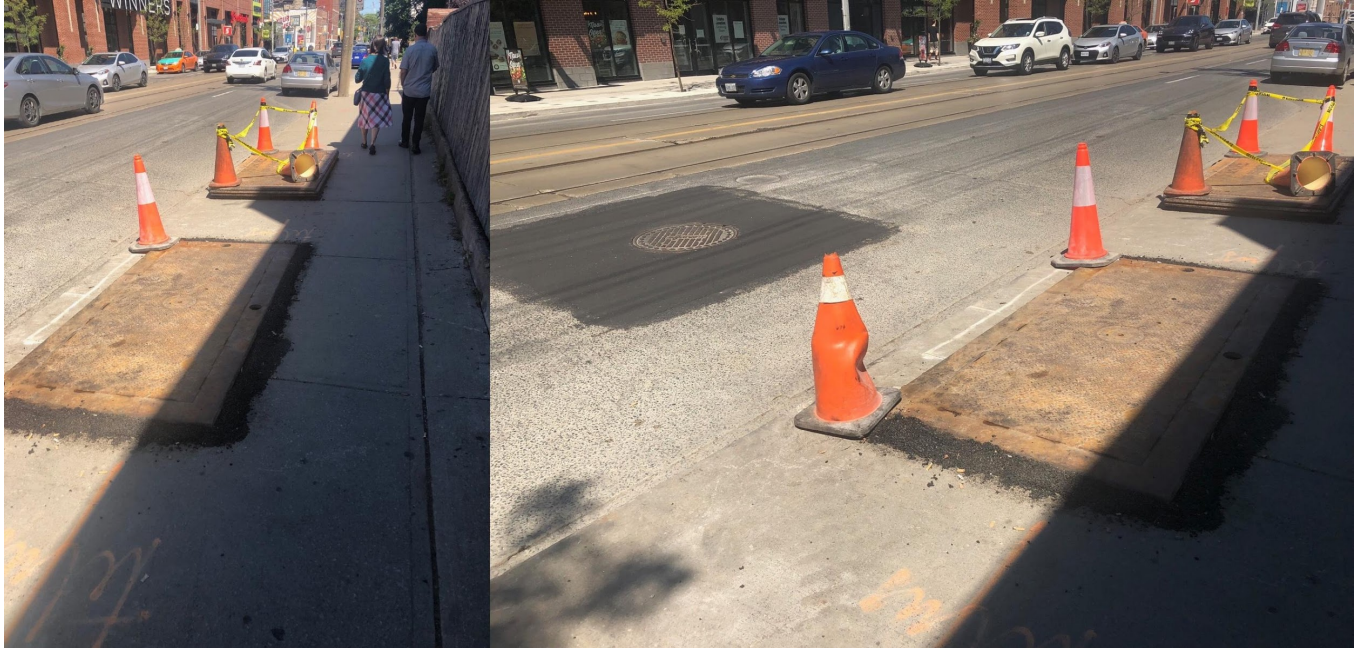
Figure 2. Installation observed to restrict access to pedestrian space. Toronto, Ontario. June, 2019.
