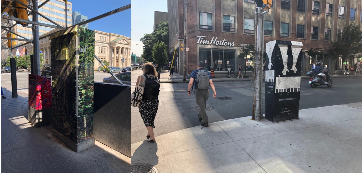
Figure 7. Above ground equipment located diagonally opposite, both pictured with aesthetic treatment. Toronto, Ontario. June, 2019.
