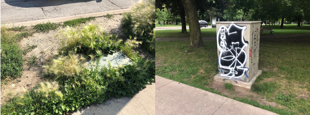
Figure 9. (Left) Grade level equipment is camouflaged by natural overgrowth and weeds. (Right) Above ground equipment covered in graffiti vandalism. Toronto, Ontario. June, 2019.
