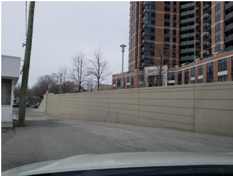
Figure 25: 403 Keele Street, showing large wall limiting view of a POPS
