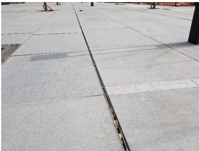
Figure 9: 8 Eglinton Avenue East POPS- April 22 Showing uneven surface tiles
