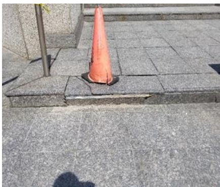
Figure 2: 1910 Yonge Street POPS – April 22 Showing broken outdoor floor tiles
