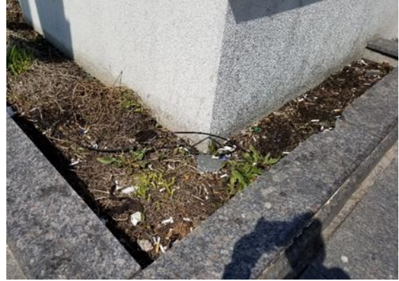
Figure 3: 1910 Yonge Street POPS – April 22 Showing garbage in planters
