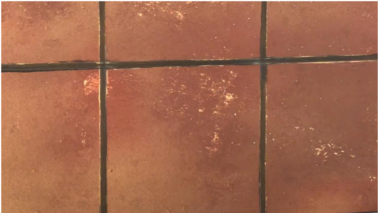
Figure 17. Close up of Tile Paint treatment, Aaron Kelly, 2018.
