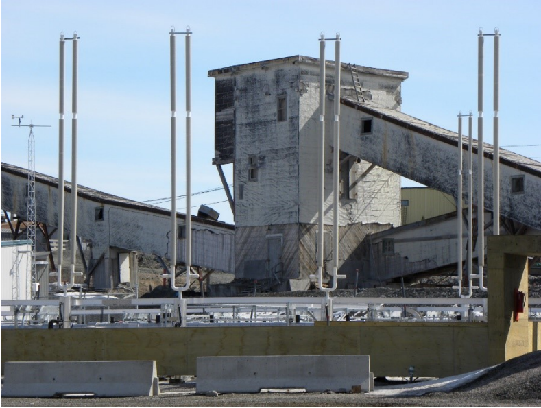
Figure 9: Thermosyphons in a test plot at the Giant Mine site. Hundreds of thermosyphons will be installed to ensure the underground chambers remain frozen.
