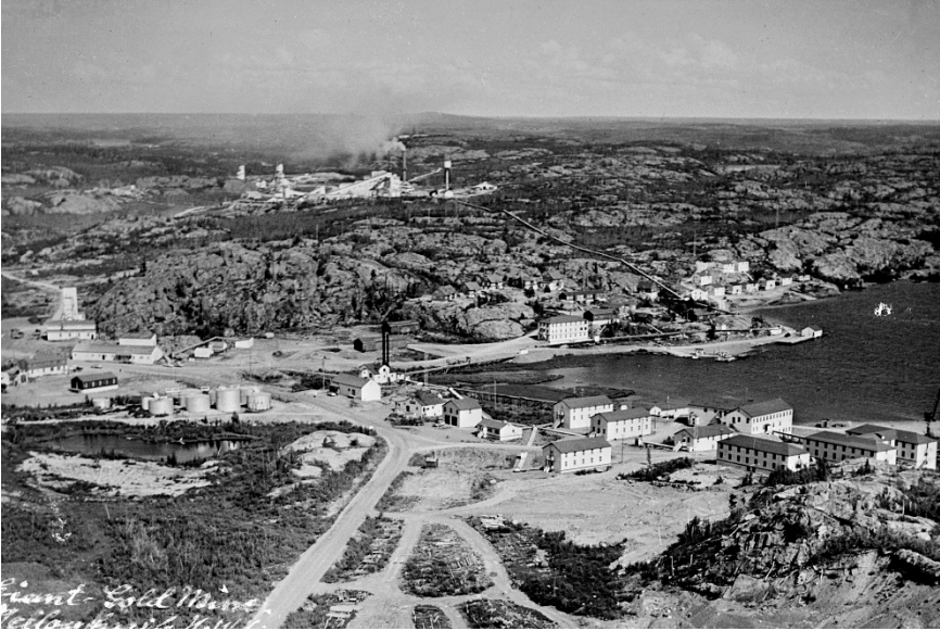
Figure 8: Aerial view, Giant Yellowknife Mine headframe and buildings nearby, 1955.
