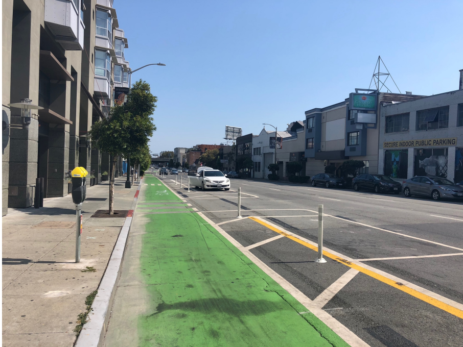
Figure 3: 7 th Avenue, looking south from Howard Street to Folsom Street. SF Transformation installed bollards along this stretch in June 2017. The SFMTA removed the bollards, and later replaced them with new ones. September 3, 2018.
