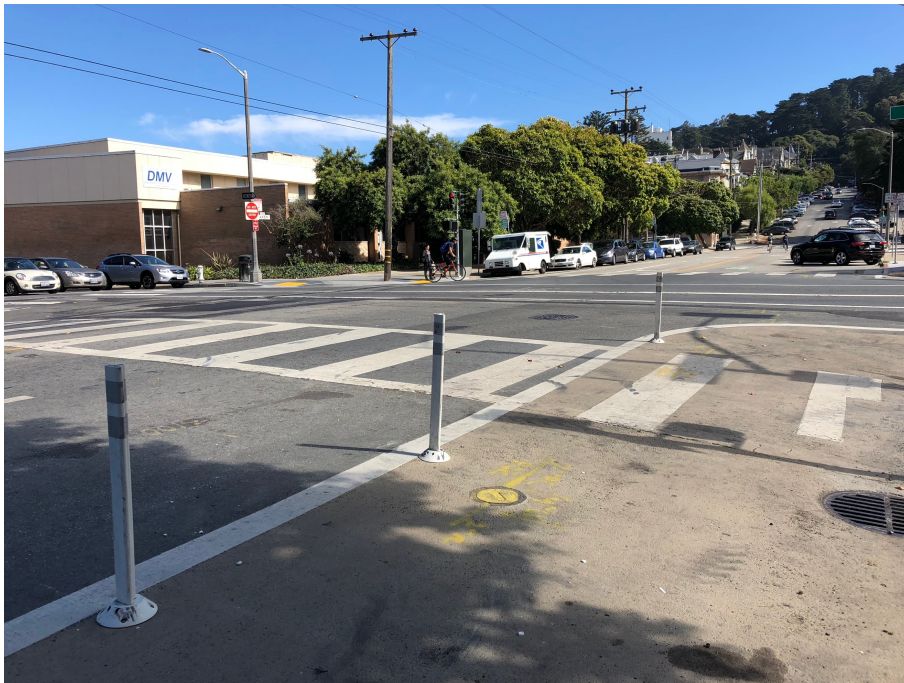
Figure 2: The intersection of Fell and Baker streets, showing the SFMTA-installed bollards that replaced the SF Transformation bollards, which were closer together and more numerous. September 3, 2018.
