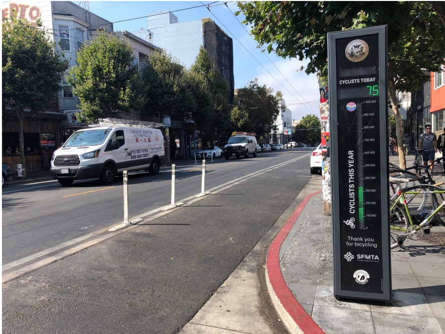
Figure 5: Three bollards installed on Valencia Street by the SFMTA, next to a bike counter monitoring cyclist activity on the corridor. September 3, 2018.
