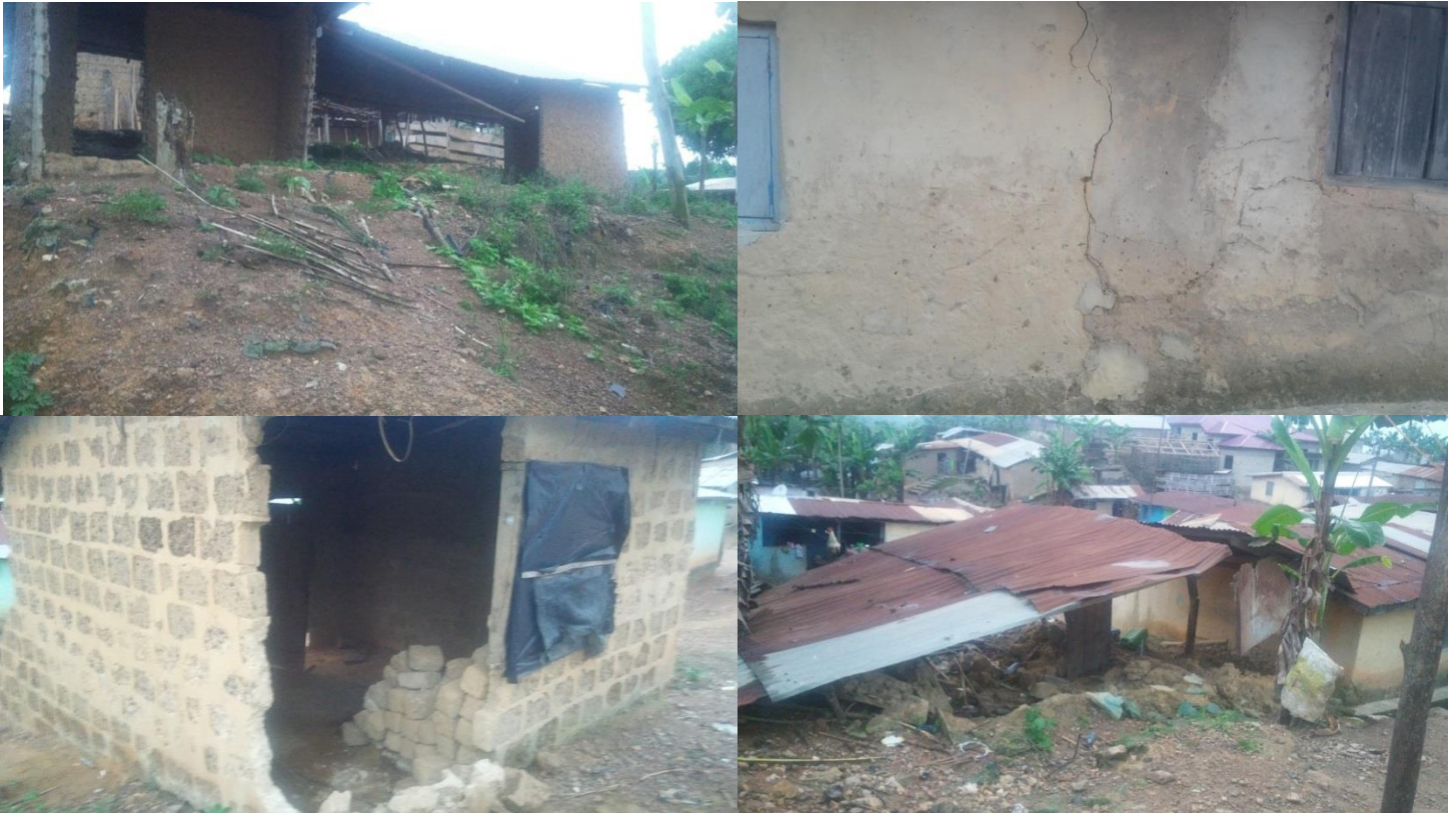
Figure 8: Cracked and collapsed or unfinished houses in Dumasi
