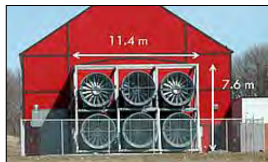
Figure 1. Controlled Wind Facility fans
