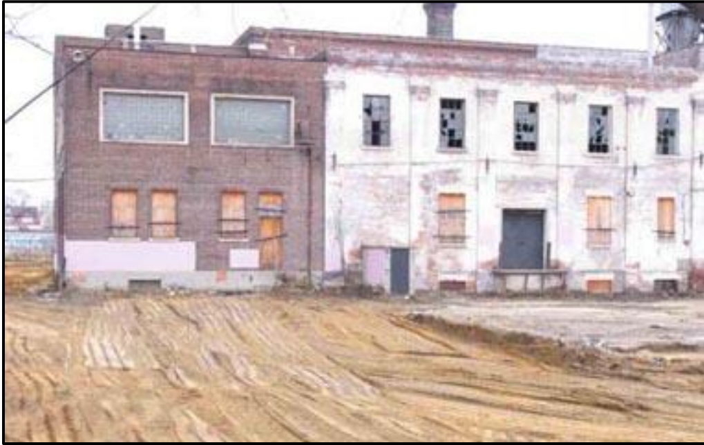
Figure 6: Remediation Activities The Fieldhouse, Sorauren Town Square and Linseed Oil Factory were remediated in 2004.
