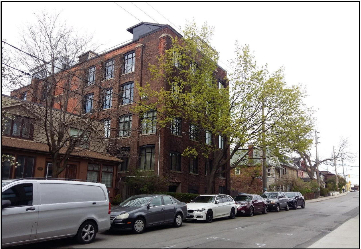
Figure 27: Low-Rise Apartment Building Low-rise apartment building on Sorauren Avenue. (Photo taken on Sorauren Avenue looking south-east).
