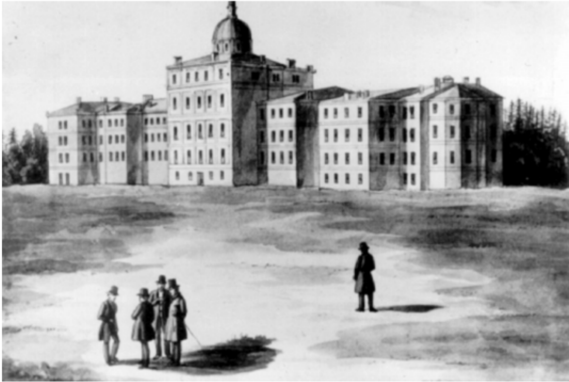
Figure 14: “Building the Asylum”
