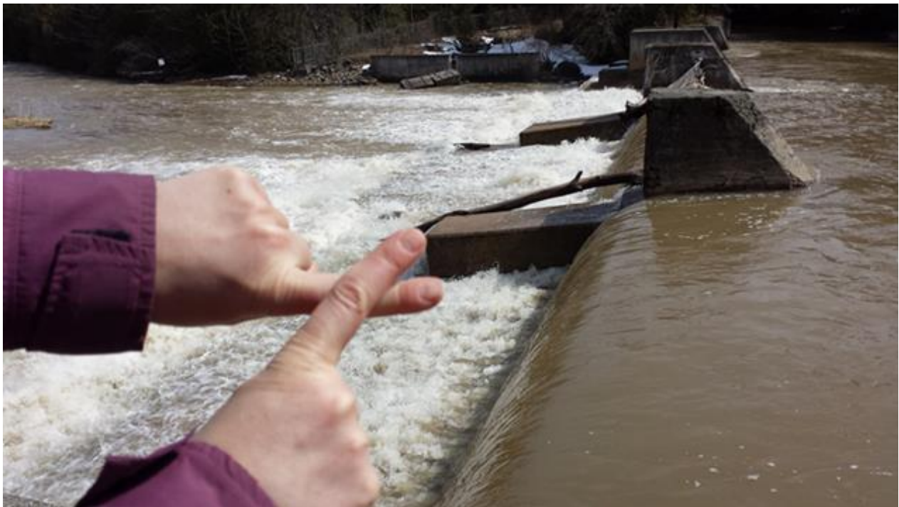
The Haines Dam in Clarksburg is in very poor shape and may have to be removed.
