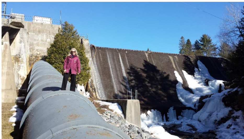
Minden generating station and Dam. Orillia Power Corporation.
