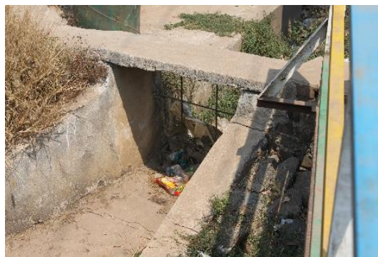
Figure 6: Waste beginning to pile up against a drainage canal grate.
