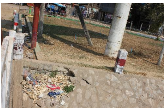
Figure 4: Damaged levee near main road.
