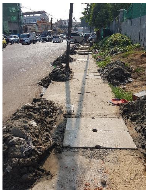
Figure 8: Drainage canal being dredged by hand.
