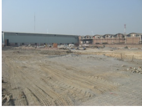
Site for extension for treatment plant
