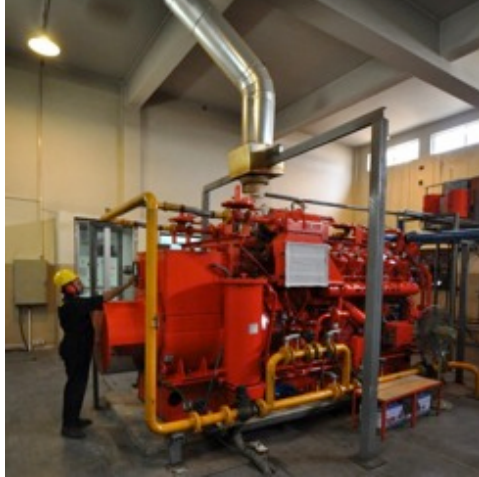
Waukesha natural gas generator
