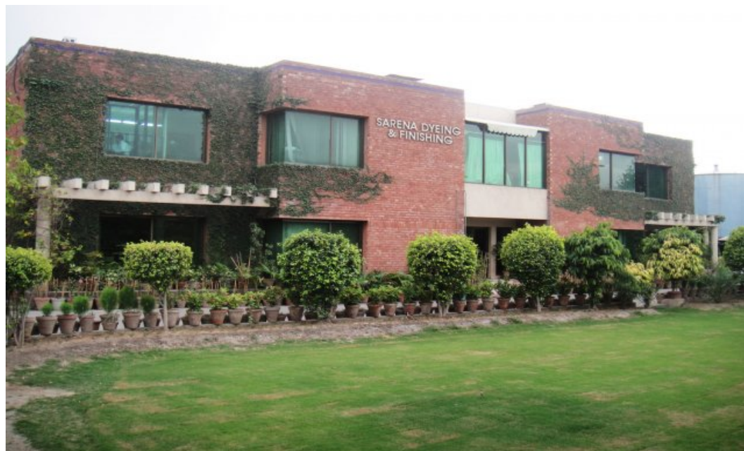
Sarena Dyeing & Finishing: Administration Block
