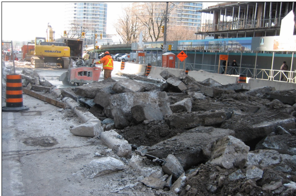
Figure 10: Queens Quay West Construction Source: Ulla Congress, used with permission
