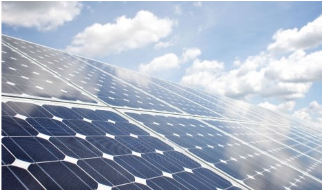
Power plant - Photovoltaic
