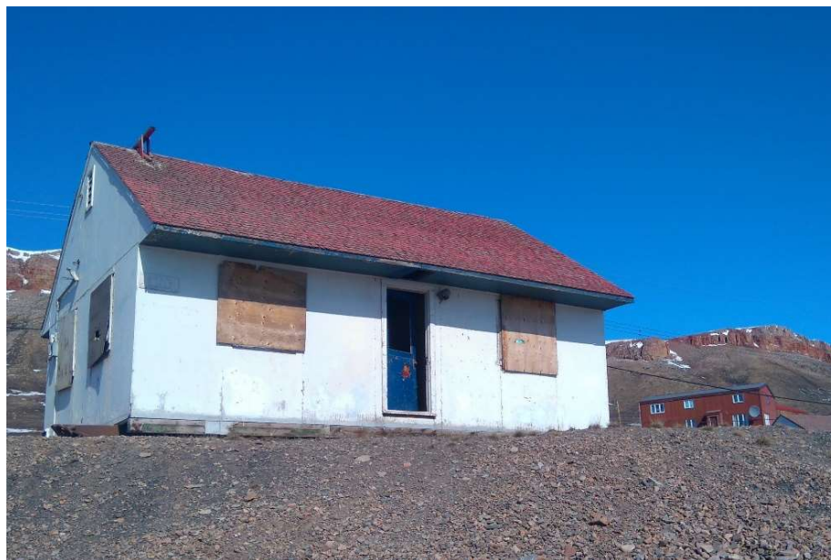
Figure 8: The original Weather Station (built in the 1940s), which later became a RCMP detachment is one of the oldest buildings in Arctic Bay. Photo taken June 2017. Sadly, it was destroyed by fire in September 2017.
