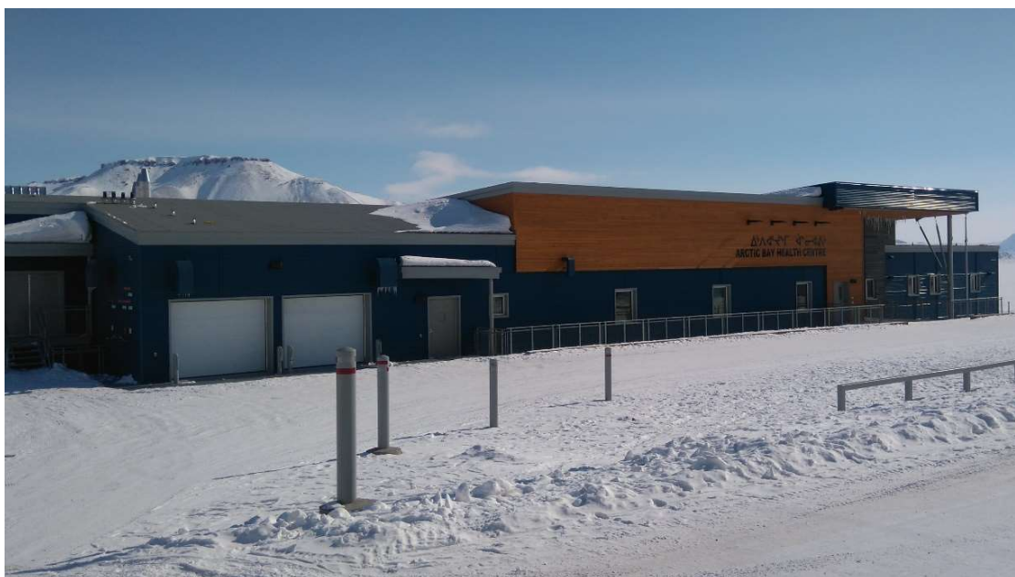
Figure 9: Arctic Bay Health Centre. Photo taken April 2017.
