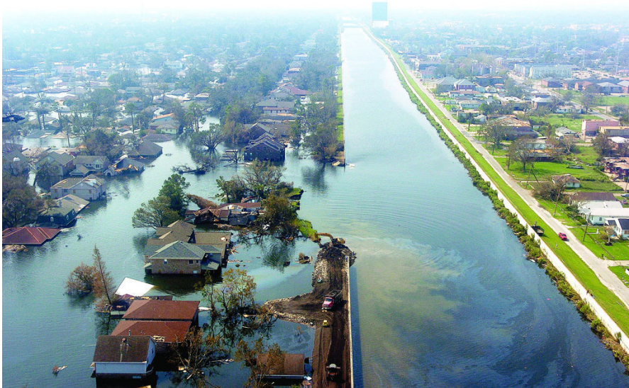
Figure 2: The 17 th Street Canal levee breached by Hurricane Katrina (Eggler, 2011).
