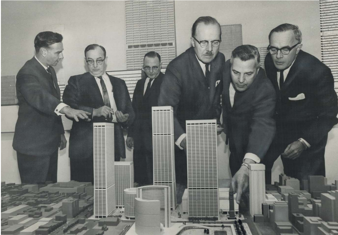
Image 3.6: City of Toronto and Metro Toronto officials, including future mayor William Dennison (with moustache) are shown a scale model of the Eaton Centre by the complex's planners, March 1, 1966. Barry Philp/Toronto Star. Toronto Public Library Baldwin Collection, tspa_0109989f.
