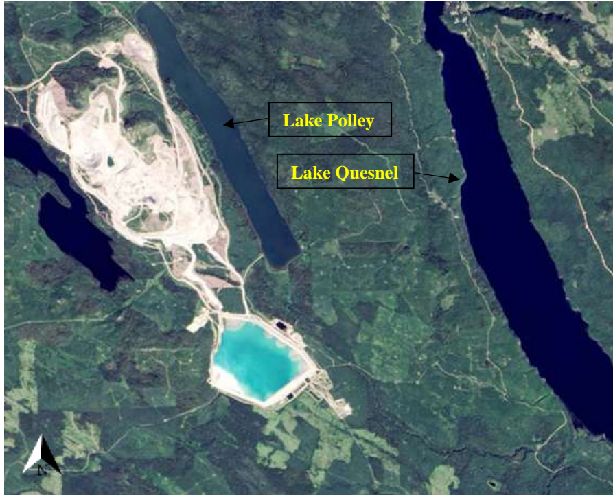
(a) Before failure on July 29, 2014
