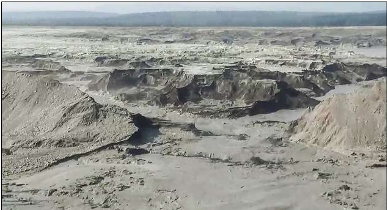
(b) Looking towards downstream
