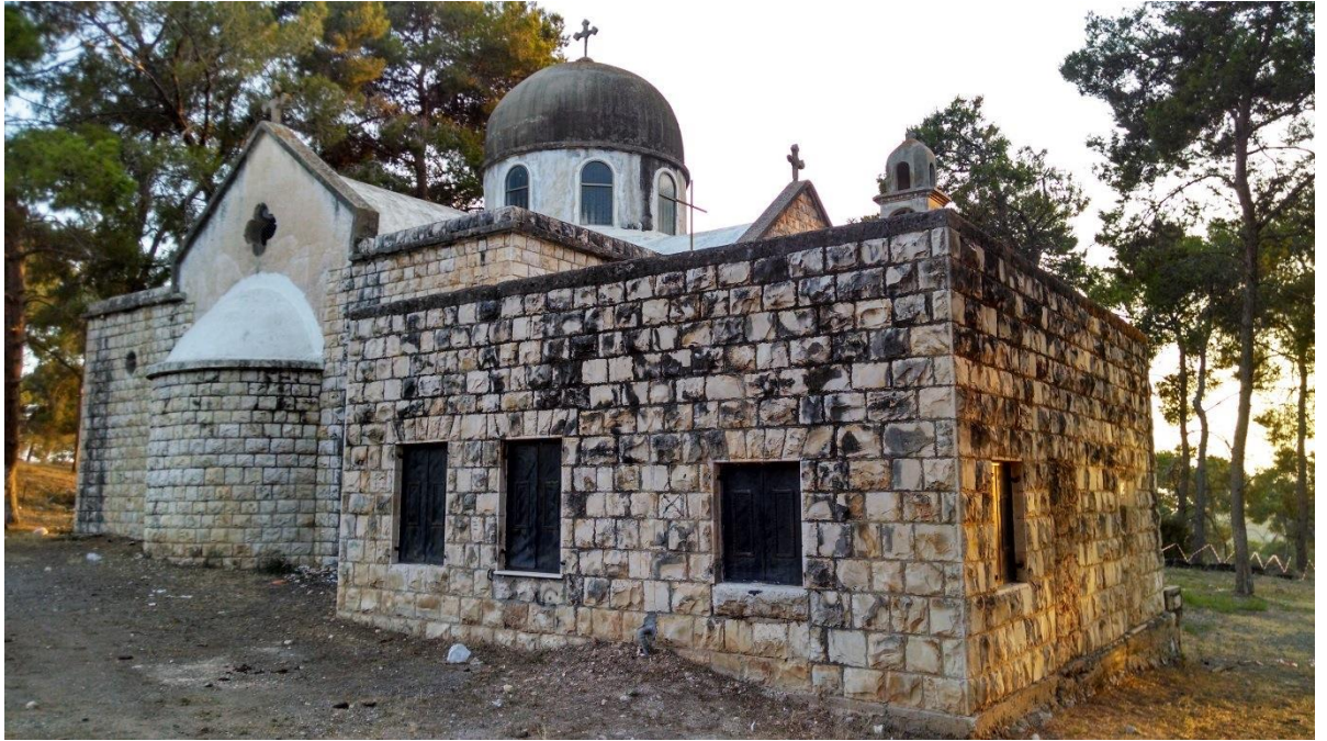
Image 38: Catholic Church of Ma'aloul cleaned and restored by Ma'aloul's families who were displaced in 1950, the last year the church served as a religious site for its dwellers before it was restored in 2011. July 2014. Photograph by the author.
