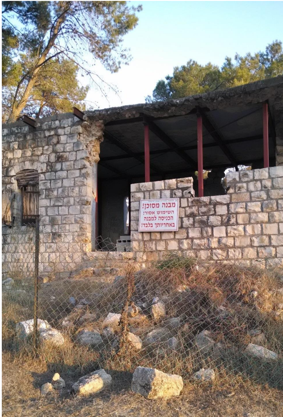
Image 37: Ma'aloul's abandoned mosque. Sign in Hebrew reads as “Dangerous Building! Using it is prohibited! Entering this building is at your own risk!” July 2014. Photograph by the author.
