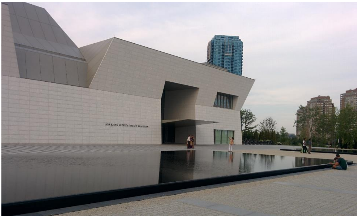
Figure 3-34. Building of Aga Khan Museum in Toronto
