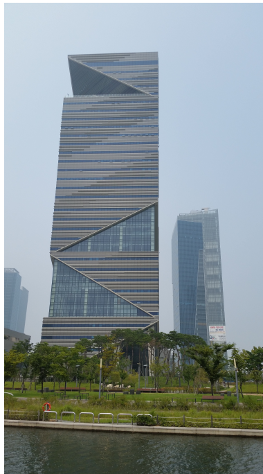
Figure 4.1 – G-Tower, IFEZ Authority Headquarters. Photographed by author’s friend (22 August 2014).
