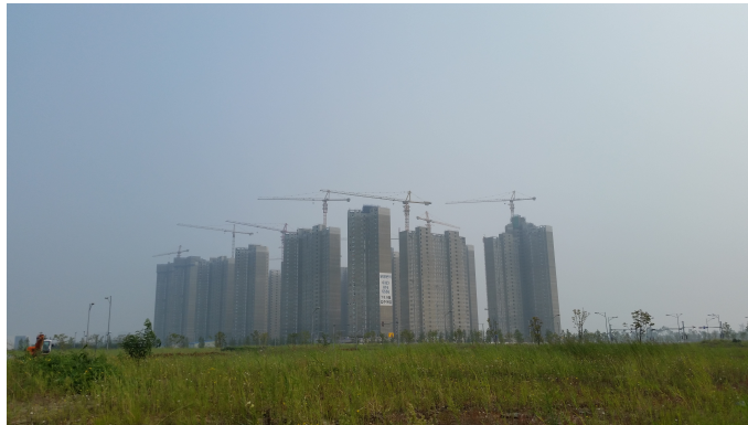
Figure 3.4 – POSCO apartments under construction in section three. Photographed by author’s friend (22 August 2014).
