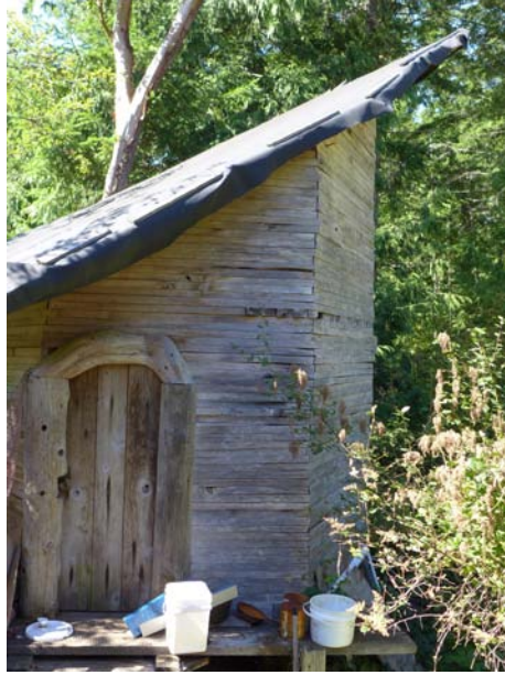
Figure 35: This construction method, of stacking 2x4s on top of each other to build a wall was a classic technique in the gulf islands during the 1970s when there was so much lumber that people were practically paid to take it off the wharfs. People would stack up their walls and then cut their doors and windows out with chain saws.
