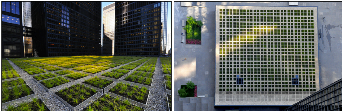
Figure 14: View of the TD Banking Pavilion green roof in Toronto. Green Reason 2014
