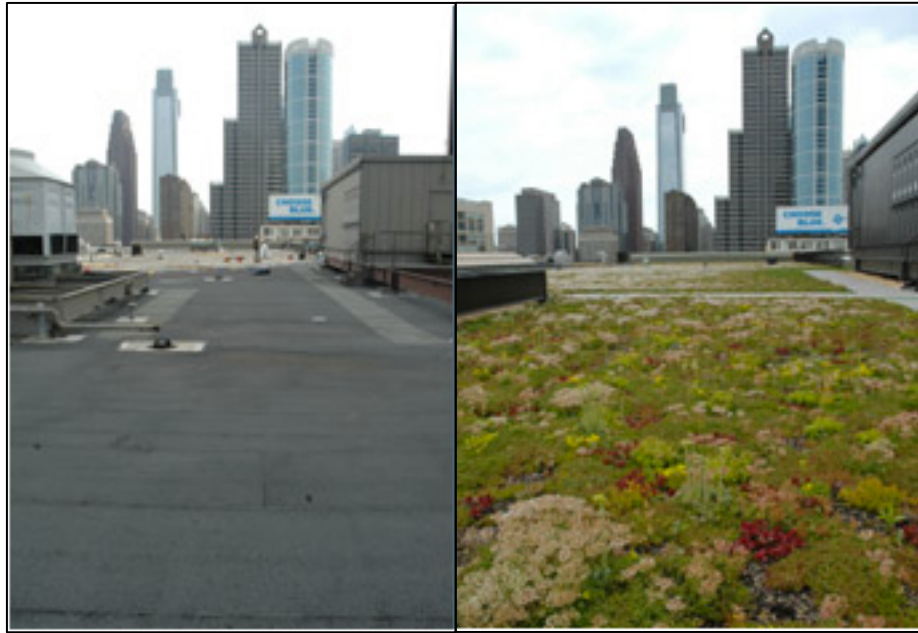
Figure 4: Before and after comparison of 45,000 square foot roof converted to green roof in Philadelphia. PECO 2009
