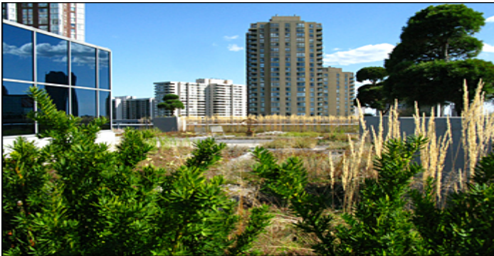
Figure 9: Intensive green roof at ESRI Canada Ltd., 12 Concorde Place. City of Toronto 2014
