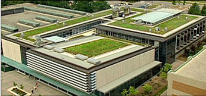
Figure 7: Extensive green roof on the Computer Science Building at York University. City of Toronto 2014
