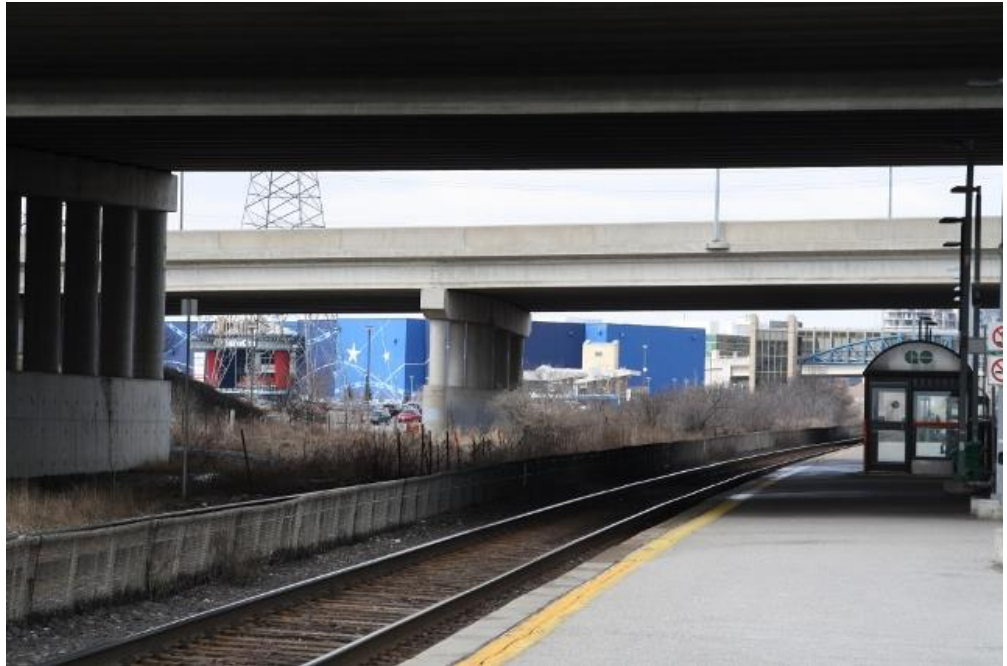
Figure 32 - The future transit concourse where the CNR tracks pass under the highways, looking from the existing GO station to the final subway station, where the existing movie theatre can be seen. The YRT bridge over the tracks can also be seen on the right. (Author photo)
