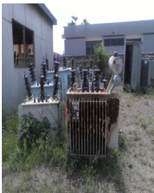
Figure 8 Pictures of PCBs tainted transformers at the ECG training School, taken during fieldtrip to the site in February 2014.
