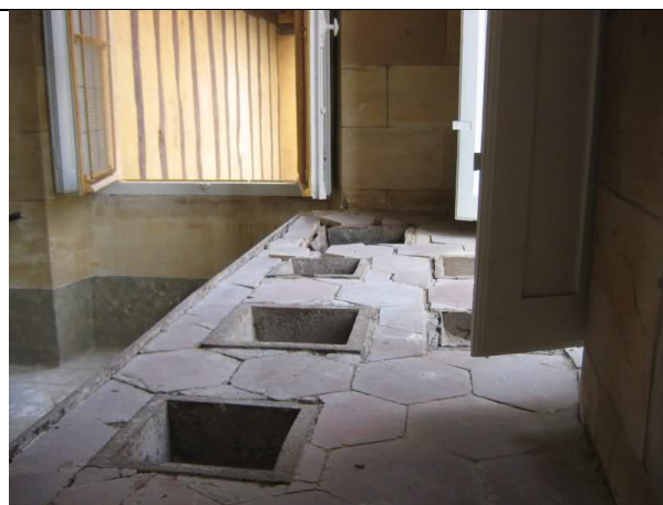
Original stove of the réchauffoir (c.1780s) of the Hameau de la Reine , Versailles. 271 I include this as an example of how little stoves changed over time between France and England. Some structures of the Hameau did not survive the Revolution, but the réchauffoir was banal enough to have avoided revolutionaries' attention (personal photograph).
