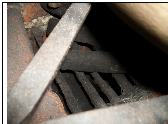
Interior of a normal stove fuel pit, this one from a stove in the main kitchen at Hampton Court Palace, London. An iron grate allows fuel to stay in place near the cooking vessel, while ash falls through the grate, for removal from the front of the stove (personal photograph). 270
