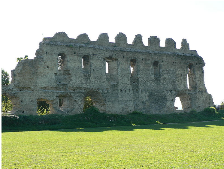
North wall of the château de Beauvoir-en-Royans, Rhône-Alpes, constructed by Humbert II.
