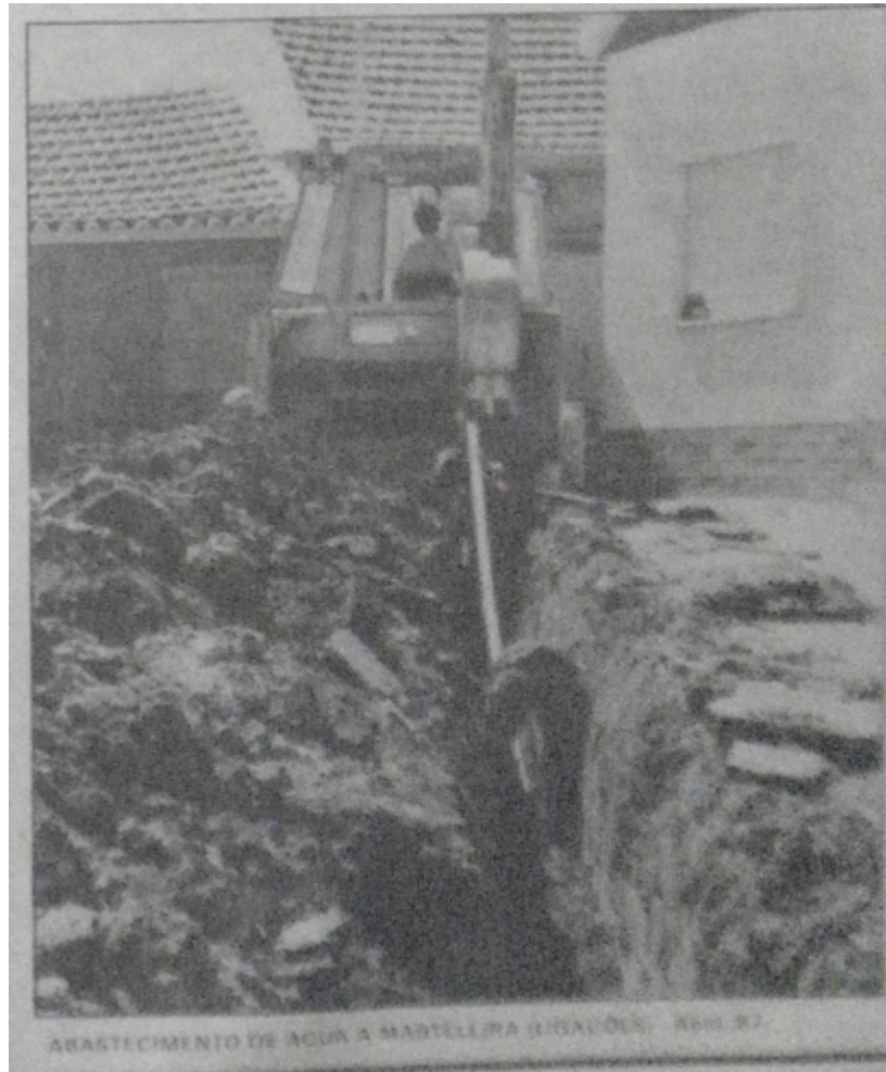
Figure 21: Digging a trench for water infrastructure, 1987. In this photo, a mechanical digger digs a trench for piping. One will note the proximity of the equipment to existing houses, highlighting the advanced residential network around which basic infrastructure needed to be installed. See: "Informação Municipal", no. 2. Alvorada (January 1987).
