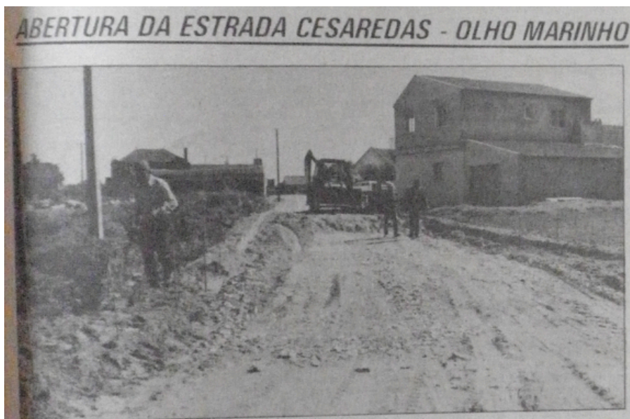
Figure 20: Lourinhã road construction, 1987. This image comes from the Municipal bulletin printed with every issue of the Alvorada in the late 1980s. A prominent feature of these bulletins was the front-page images of infrastructure improvements from across the Concelho. See: "Informação Municipal", no. 2. Alvorada (January, 1987).
