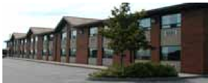
Fig.1 Peel Family Shelter
