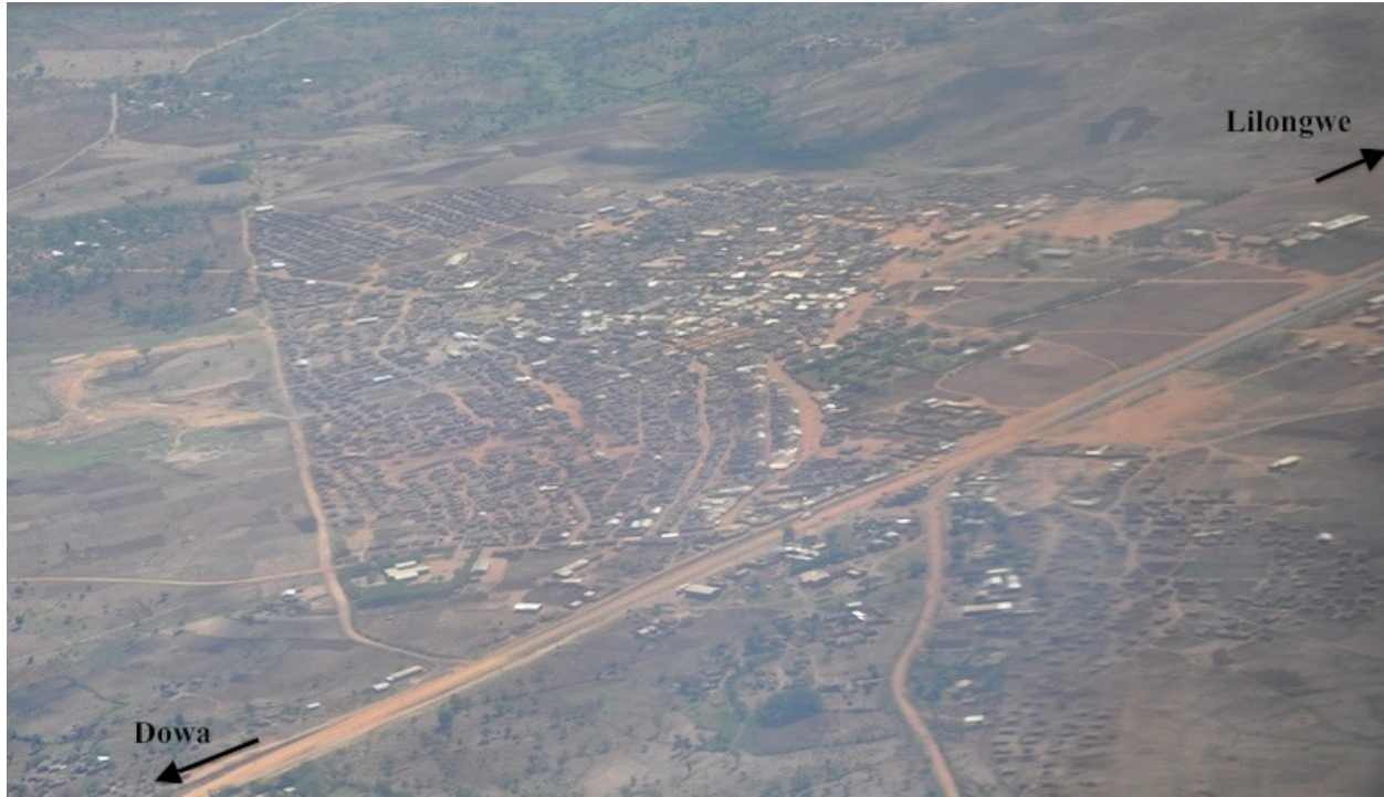
Figure 1.3: An aerial photo of Dzaleka Refugee Camp, showing the orientation of the camp towards the capital city, Lilongwe and nearest town, Dowa. Photo courtesy of Patrick Garety (2013); labels added by author.
