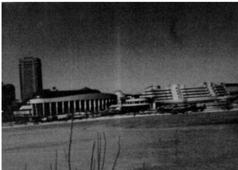
FIGURE 2: The Canadian Museum of Civilization, Hull, Quebec under construction in March 1988.
