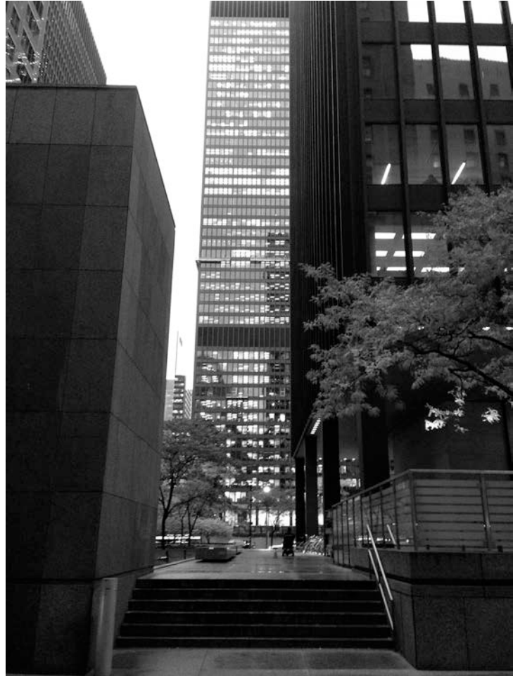
Figure 2. Toronto Dominion Centre plaza and buildings (Photograph by author).
