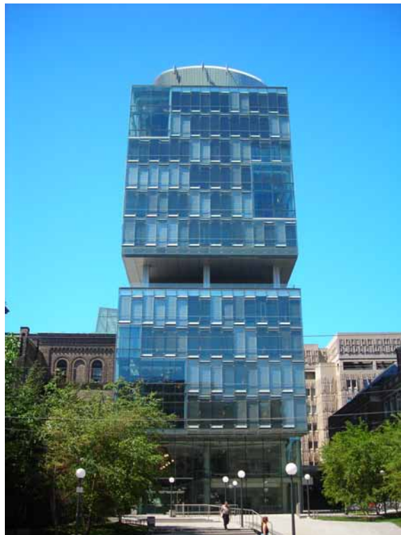
6.2. Façade of the Terrence Donnelly Centre for Cellular and Biomolecular Research (CCBR), as seen from College Street.
