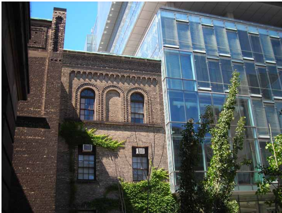
6.4. Adjacent façades of the CCBR and Rosebrugh Building.
