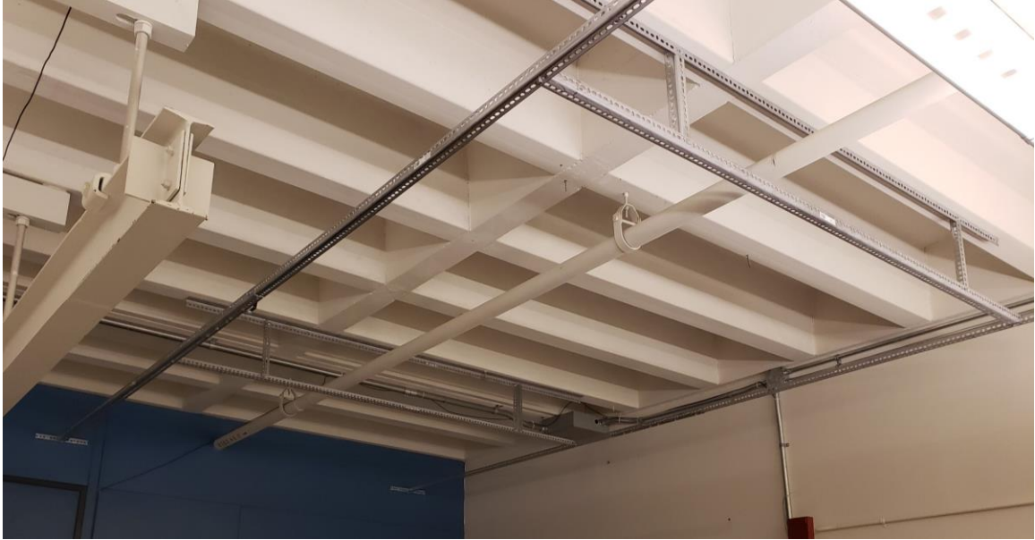
Figure 3.12 - Star Field Support Scaffolding
