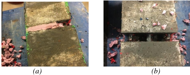
Figure 4-28 (a) Removal of the foam board and (b) extension of the auxiliary bars
