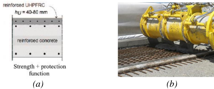
Figure 1-7: (a) Chillon Viaducts UHPC reinforced bridge deck design (b) and application (Sritharan et al. , 2018)
