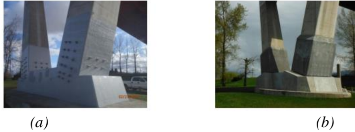
Figure 1-6: (a) Bridge pier prior (b) and after retrofitting (Doiron, 2017)
