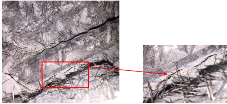
Figure 5-49 Shape of the concrete in between the ribs (Beam IE1C1 – A)
