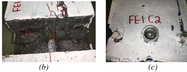
Figure 5-32(a) Crack pattern of cover after failure, (b) pullout of the bar and (c) slip of the bar
