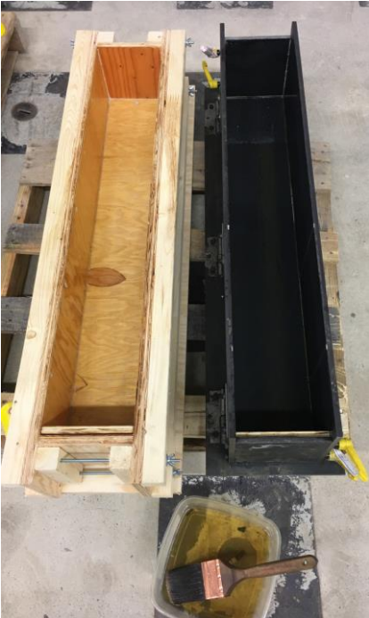
Figure 4-6 Oiling of the wood and steel formwork
