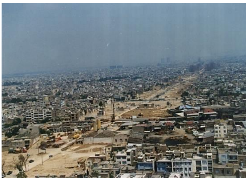
Figure 18: Neighbourhoods demolished to widen the Navab Street
