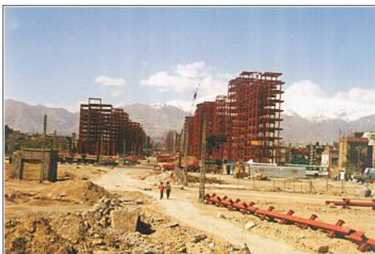
Figure 19: Navab construction site 1994
