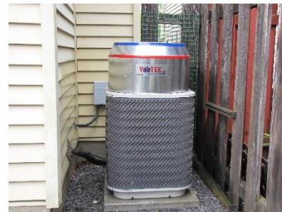
Figure 1. Typical installation of a VairTEX Air Director on top of residential condenser unit
