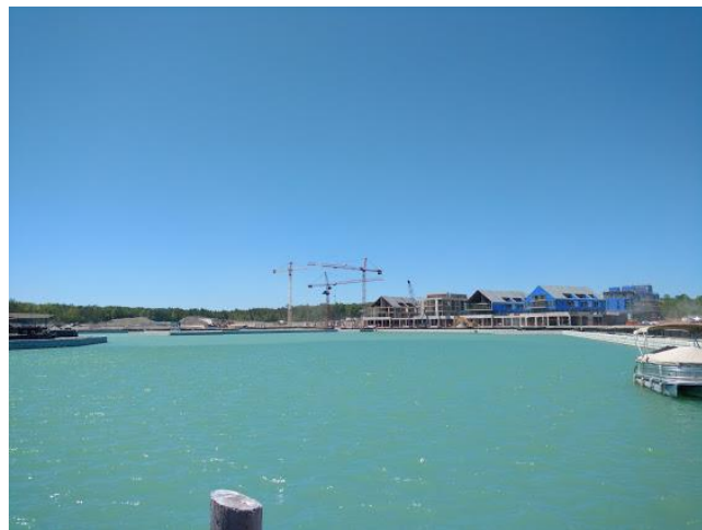
Figure 12. Flooded Marina, Friday Harbour Development Site
