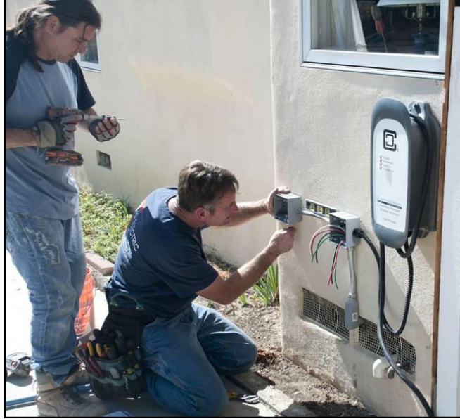
Figure 23: Connecting Electric Vehicle Charging Station to the Electrical Rough-in (Paul Gipe, 2014)
