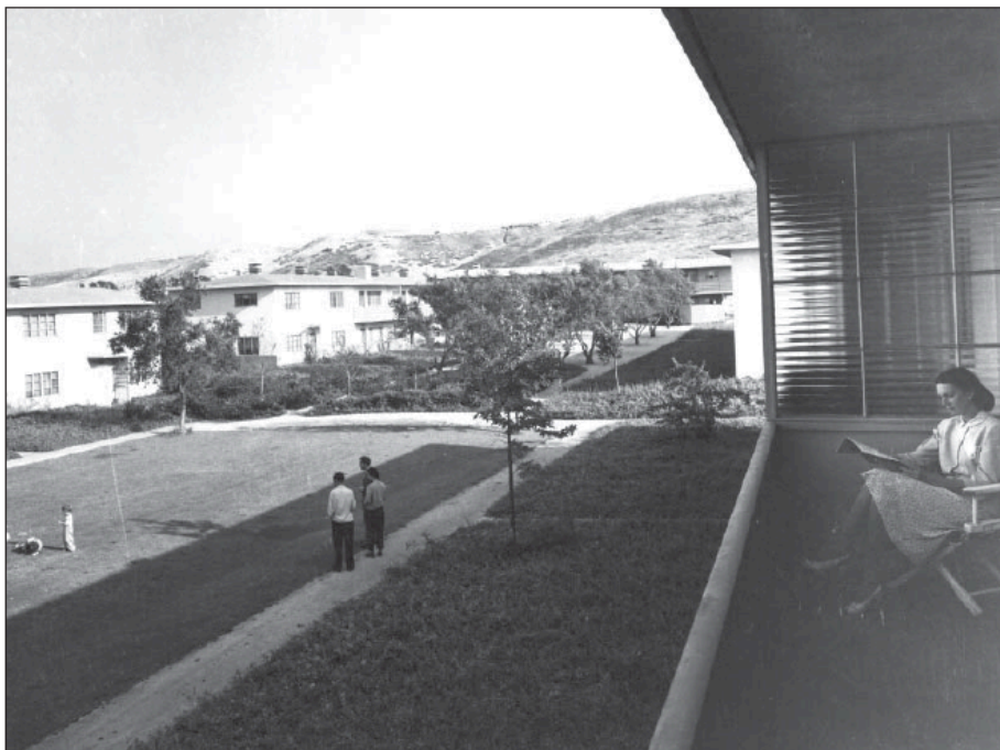
Fig. 13: Baldwin Hills Village, Baldwin Hills, California, 1942. Reginald D. Johnson, Robert Alexander, Lewis Wilson, Edwin Merrill, Clarence Stein, architects. Fred Barlow, Jr, landscape architect. Source: "Garden Apartments of Los Angeles: Historic Context Statement": 55.
