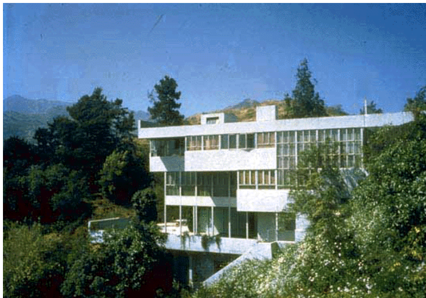
Fig. 9: Lovell Health House, Los Angeles, California, 1929. Richard Neutra, architect. Source: http://www.neutra.org/tours.html
