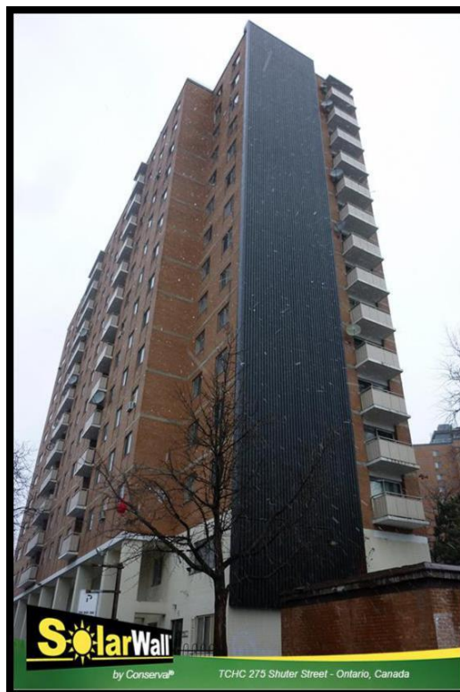
Figure 6.1 - Pictured is a SolarWall© located at 272 Shuter Street in Toronto's Moss Park neighbourhood. The system provides solar heated air to residents of the building which reduces the uses of natural gas.
