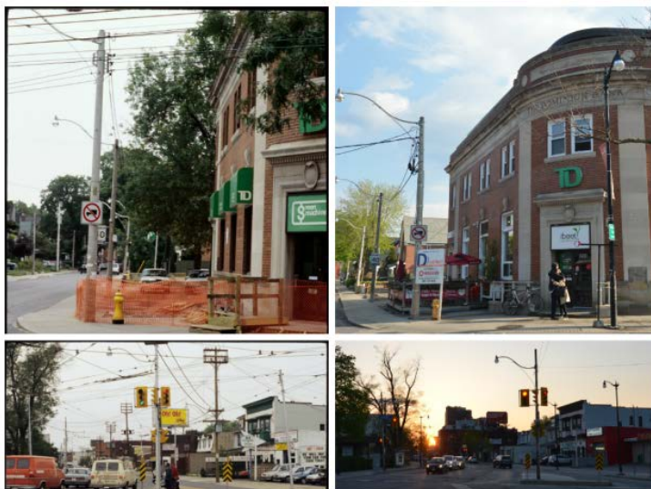
Figure 33 – These four pictures (left side is before, right side is after) show the full extent of The Junctions revitalized streetscape. Note the removed hydro lines and the new street lights that were installed.
