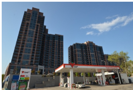
Figure 41 - Both of the Heintzman Street (formally Options for Homes) condominium towers, which are comprised of 643 affordable condominium units.
