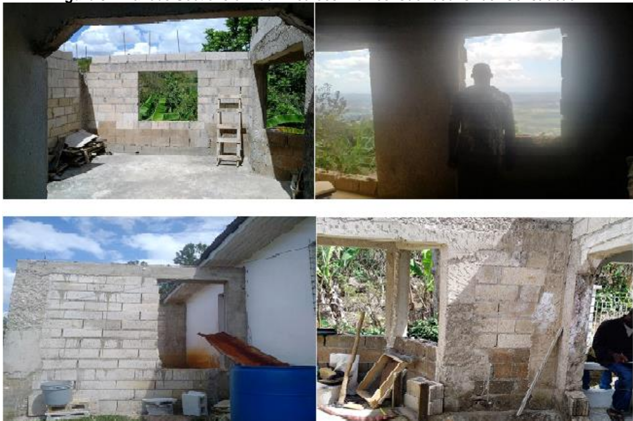
Figure 5 – Various Sections of Four ‘Retirees’ Homes ‘Stranded’ Under Construction
