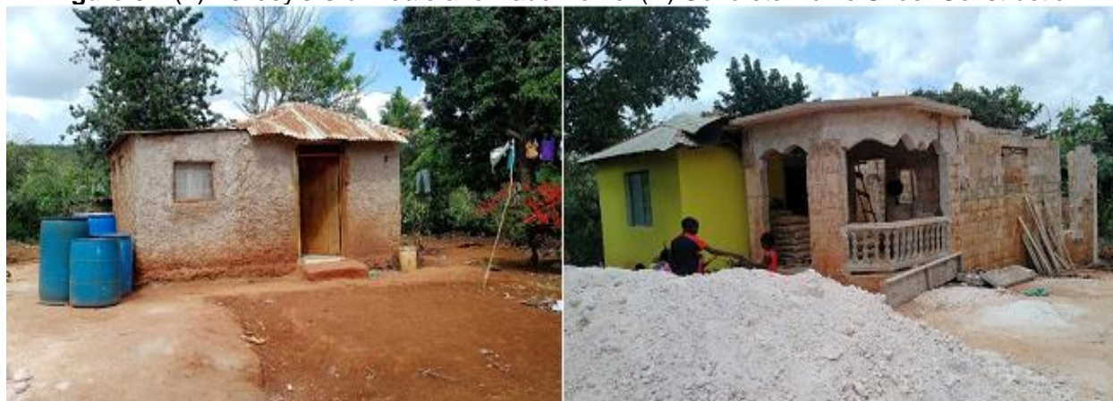
Figure 6 – (L) Bentley's Old Wattle and Daub Home. (R) Concrete Home Under Construction
