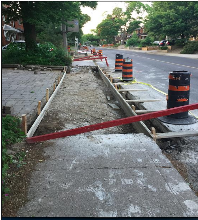
Figure 11 - Sidewalk Construction on Jedburgh Road
