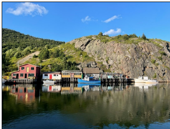
Figure 14: Example of bedrock coast with vulnerable buildings, Quidi Vidi, August 2021 (Way, 2021)
