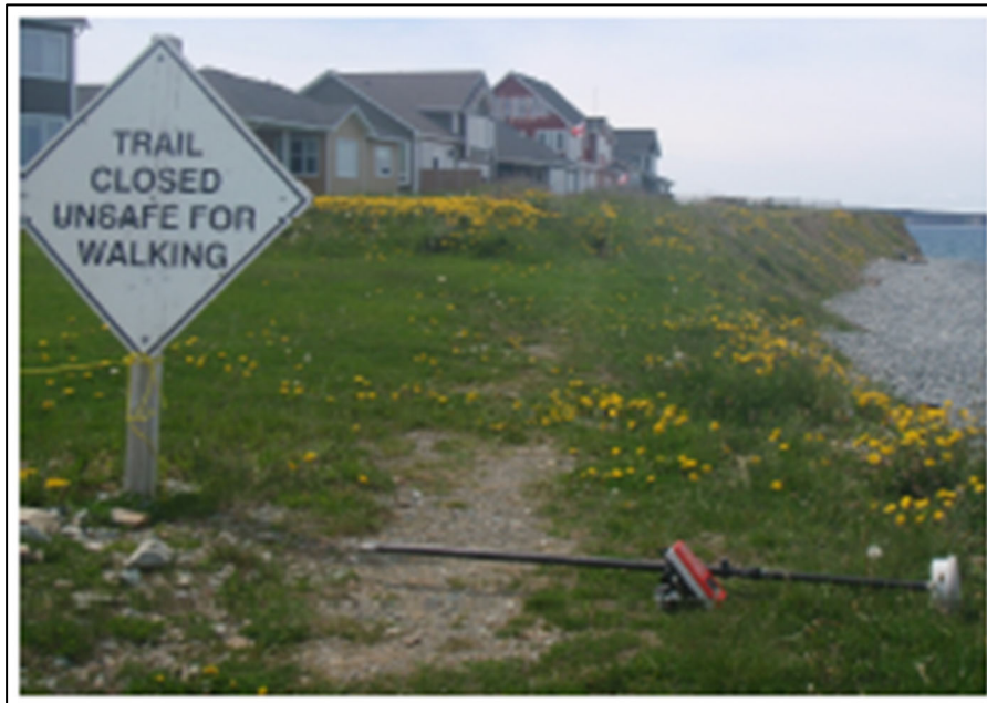
Figure 9: Closed trail due to coastal erosion (Batterson, 2020, p.9)
