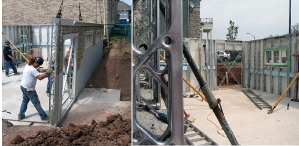
Figure 3-2 TSP panels erected on-site (“Products@www.nexcon.ca” 2011)
