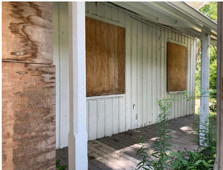
Figure 4.2: Wooden decking of the house (author's photo)
